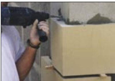
Drilling a hole for the rawlplug
